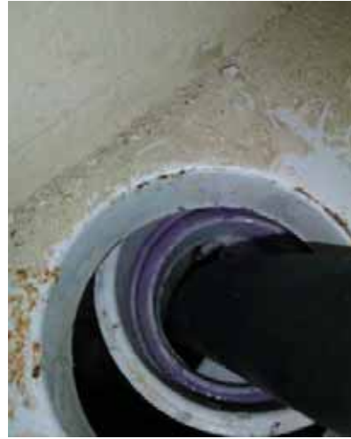
Image 10520-202. Drainpipe cement fails; drainpipe becomes detached from washing machine water supply box.
