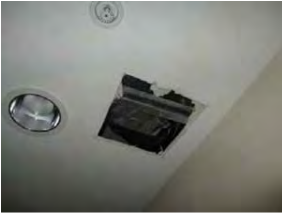
Plumbing Repair Holes in Ceiling, Unit 302, Below Unit 401
